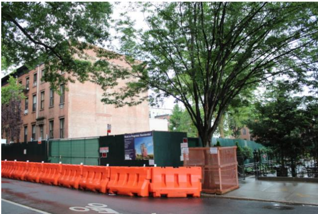
"5 River Park" has started construction recently. (Reporter Liu Daqi / Photography)
