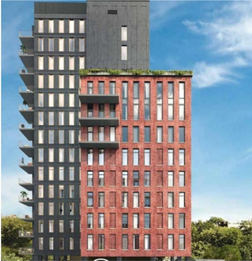
"5 River Park" has started construction recently. (taken from the official website)
